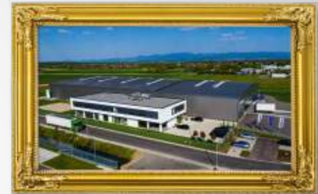
2017 New plant in Willstätt
